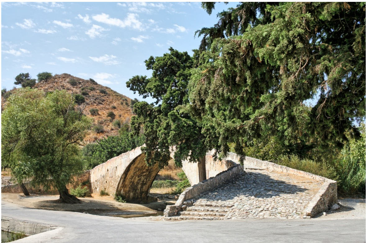
After repair – removed: person, cable, road sign, bench, fences and the energy pole.
